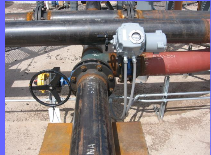
Pressure and Flow Control Valves
