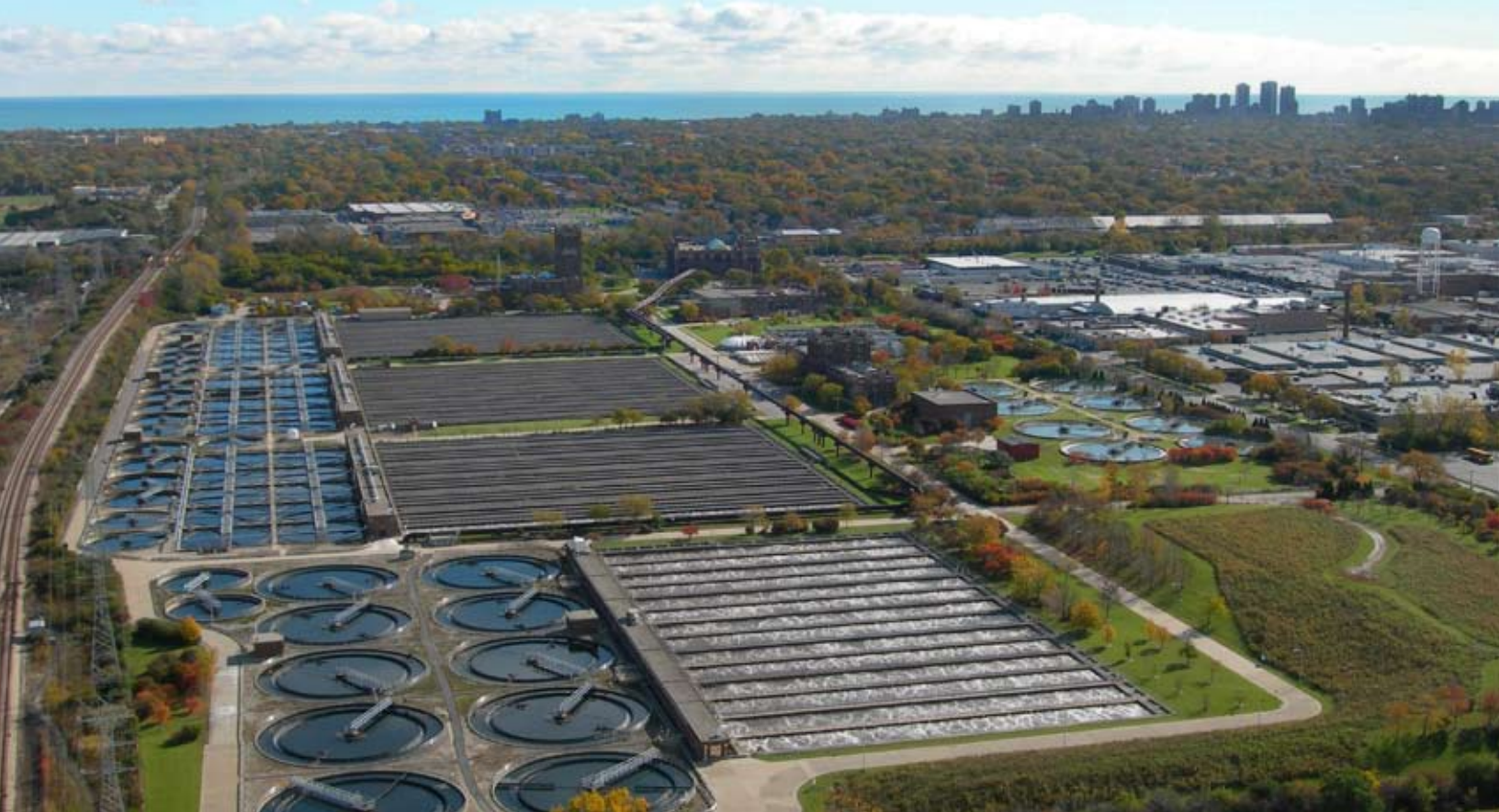
The Chicago Northside Water Treatment Plant along Lake Michigan. Photo courtesy of the Metropolitan Water Reclamation District of Greater Chicago.
