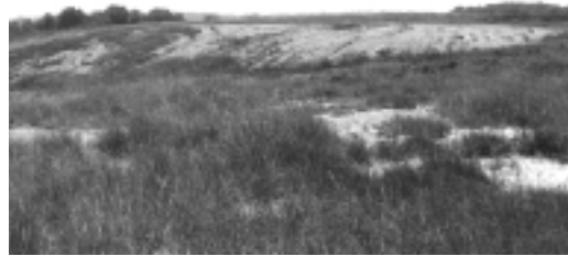
Landfill site showing gully erosion. (Photo courtesy Northeast Indiana Solid Waste Management District.)
