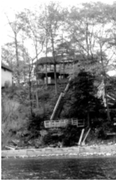
Example of Oswego River streambank erosion (Photo courtesy the Oswego County Soil and Water Conservation District.)
