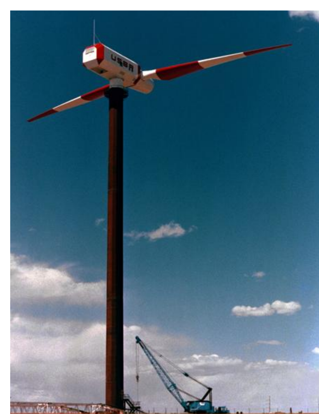
4 MW WTS-4 in 1982 (held the world's record for power output for over 20 years)
