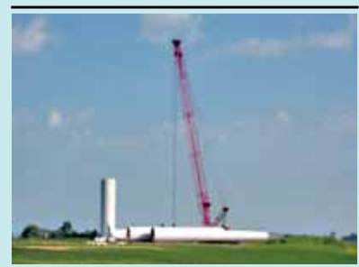
Construction of Port Alma Wind Farm, Ontario. Photo credit: Ironworkers Local 700, 2007.
