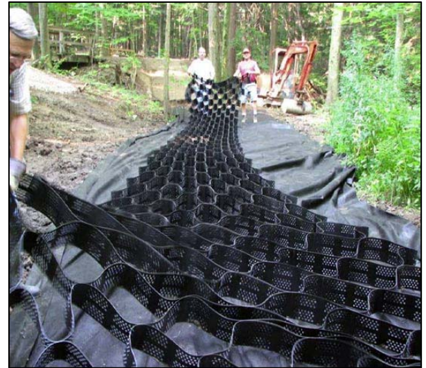
Geo-cell installation for soil erosion control. Photo: Pennsylvania State University.
