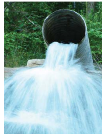
Sewer pipe, © James McQuillan.
