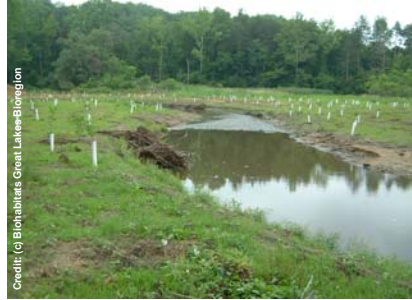
Restoration of Silver Creek in Geauga County, Ohio, conducted by the Geauga Park District. The project restored 1,000 feet of the creek, a cold water stream that supports trout habitat. The project realigned and adjusted the plan, profile and cross section of the creek, and enhanced in-stream habitat, riparian wetlands and native reforestation. The white tubes protect newly-planted trees from deer browsing.
