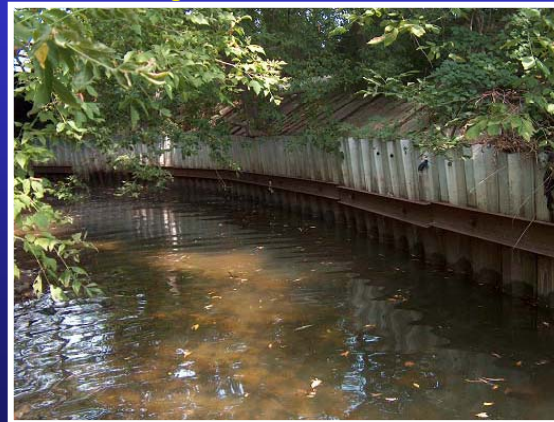
Failing Bank Protection
