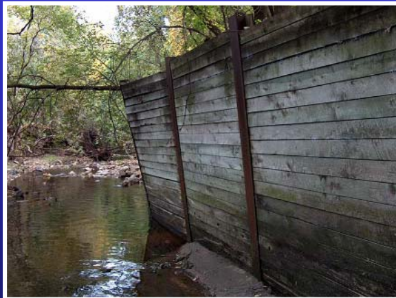
Failing Bank Protection
