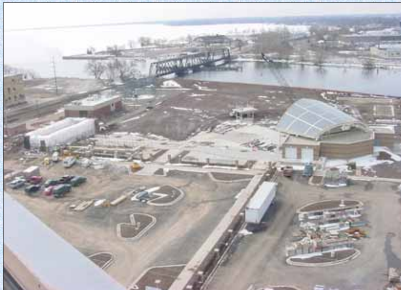
Site Currently Under Construction, 3/24/05
