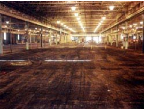
Quad/Graphics West Allis Facility
