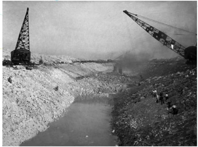
**Digging the canal** in Palos Park, Ill., in 1914. Pictured is the construction of the Calumet feeder to the drainage canal.
