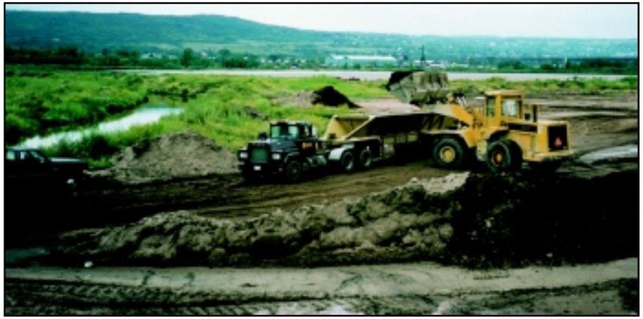
Figure 15: Construction fill being loaded at the Erie Pier Confined Disposal Facility in Duluth, Minnesota
