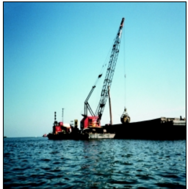
Figure 7: Mechanical dredging using a crane and barge
