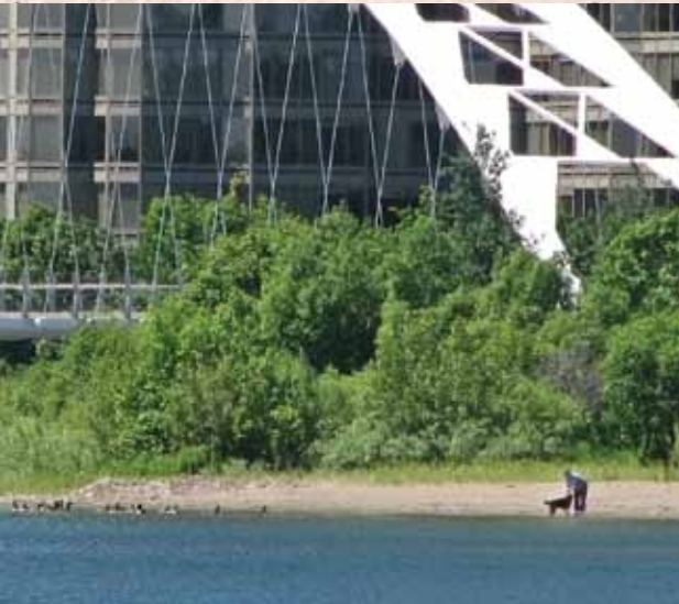
Lake Ontario Humber River Pedestrian Bridge Toronto, ON
