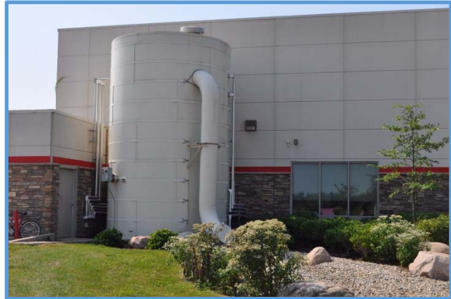
Large retailer captures roof drainage to irrigate surrounding green infrastructure
