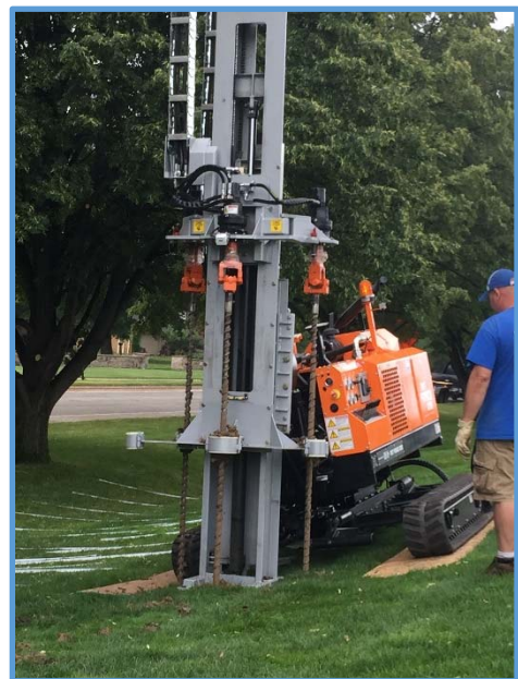
Infiltration Enhancement being installed along grassed swale
