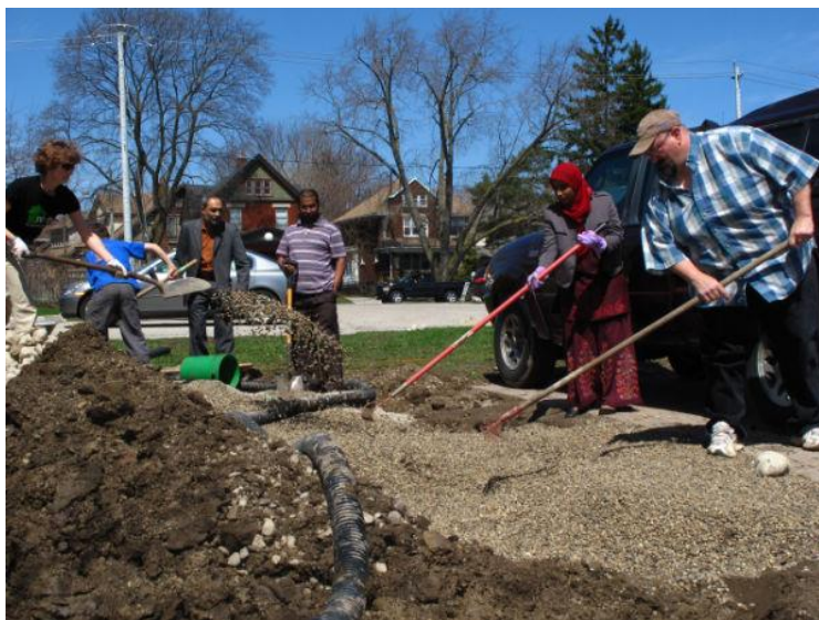
Interfaith Bridge Building rain garden construction event at REEP House 2011
