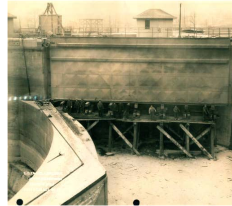
Building upper miter gates of Brandon Lock 1935 ( 2014-01-I&MCanal-0063 )
