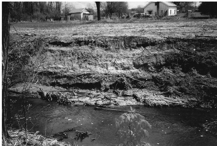
Before and after photos of a streambank restoration bioengineering project previously funded by the Great Lakes Basin Program
