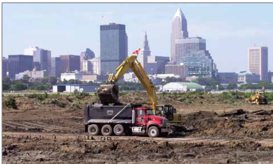
300,000 cubic yards of sediment was removed from CDF 10B in Cleveland and used to cap a 58-acre Brownfield site off Pershing Avenue. The site is slated for redevelopment as an industrial park.
