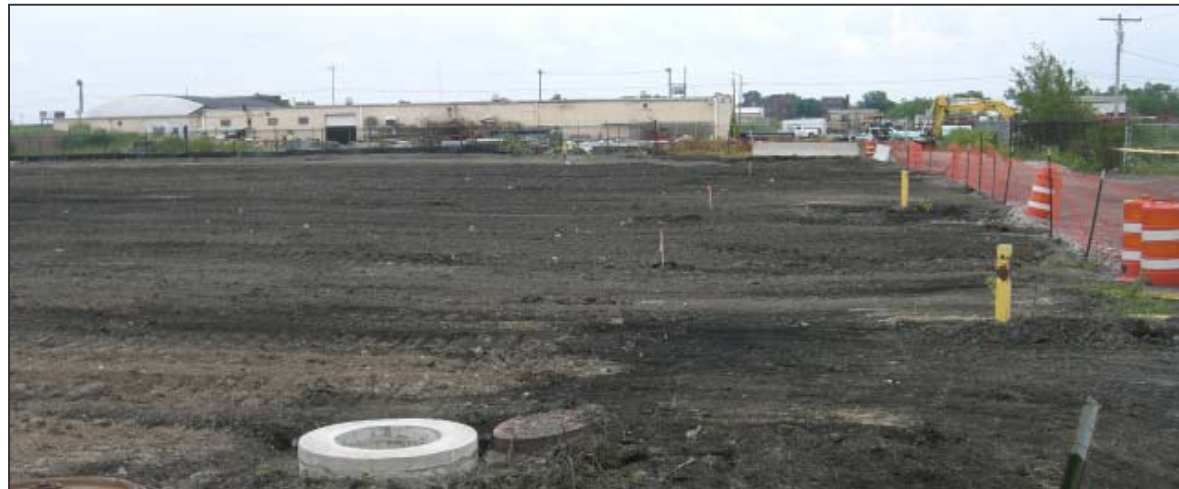
LNAPL remediation Area west of Orlando St. complete
