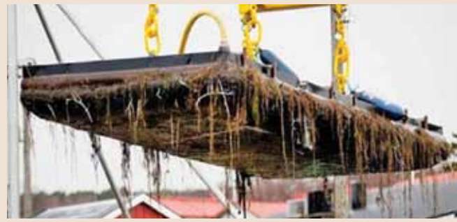
Cranes lift a slab of frozen toxic sediment at the Swedish port of Stockholm.
