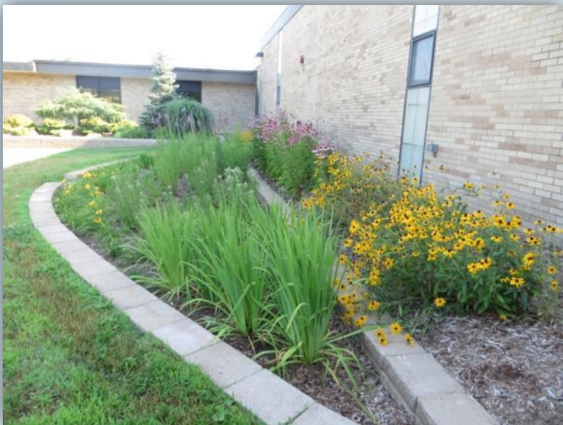
Wayland, MI – 700 SF Rain Garden installed in 2012 to intercept storm water from roof drains
