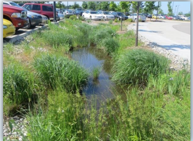
Okemos, MI – Rain Gardens and bioswales installed in 2010 to intercept storm water from parking lots and roads
