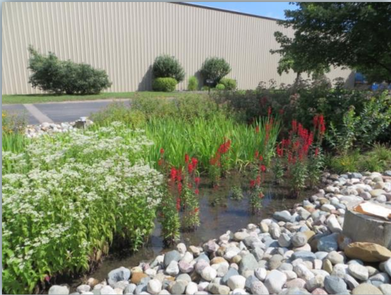
Belleville, MI – 4,600 SF Rain Garden installed in 2012 to intercept storm water from roof drain and parking lot.
