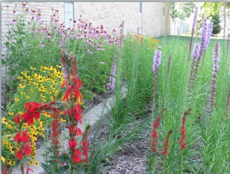
Wayland, MI – 700 SF Rain Garden installed in 2012 to intercept storm water from roof drains
