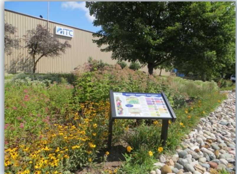
Belleville, MI – 4,600 SF Rain Garden installed in 2012 to intercept storm water from roof drain and parking lot.
