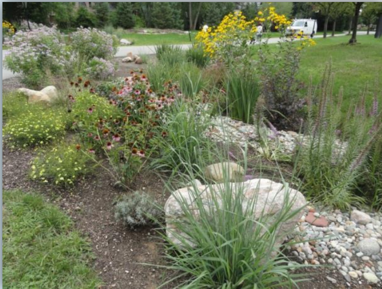
Bloomfield Hills, MI – Rain Gardens installed in 2010 to intercept storm water from road
