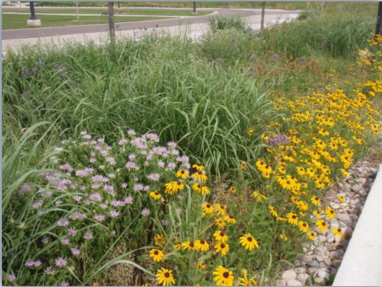
Okemos, MI – Rain Gardens and bioswales installed in 2010 to intercept storm water from parking lots and roads
