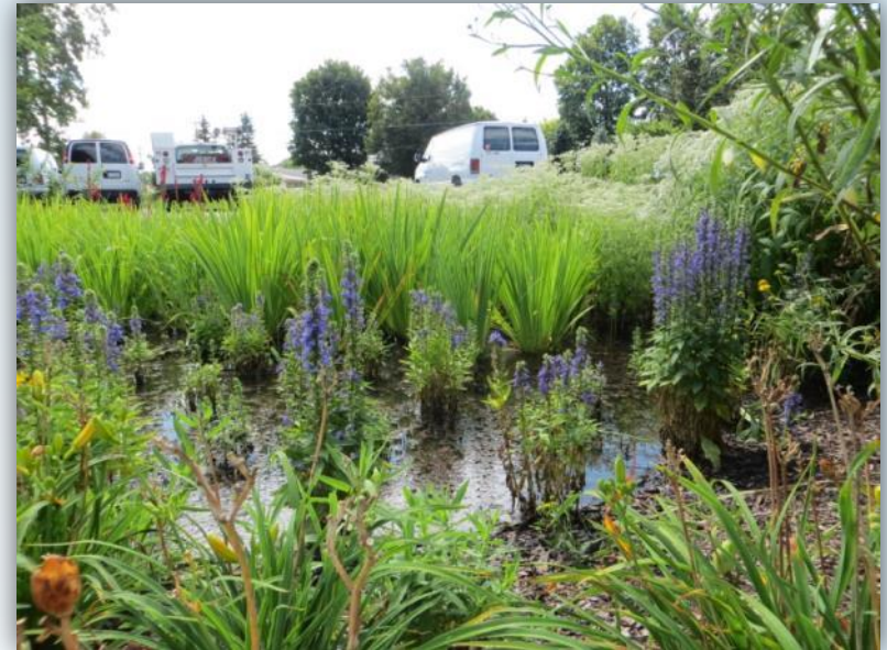
Belleville, MI – 4,600 SF Rain Garden installed in 2012 to intercept storm water from roof drain and parking lot.
