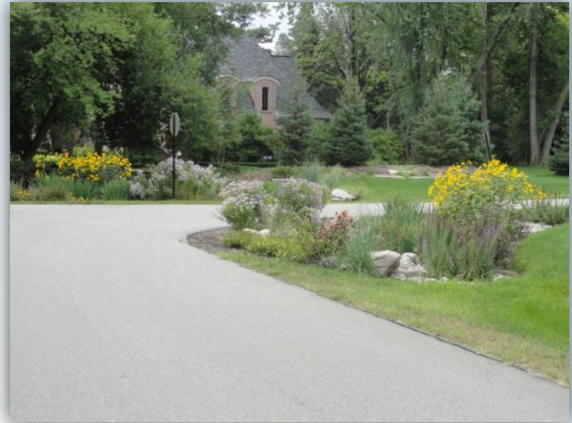
Bloomfield Hills, MI – Rain Gardens installed in 2010 to intercept storm water from road
