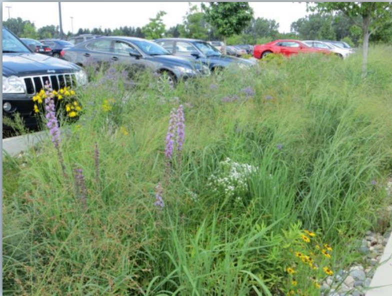
Okemos, MI – Rain Gardens and bioswales installed in 2010 to intercept storm water from parking lots and roads
