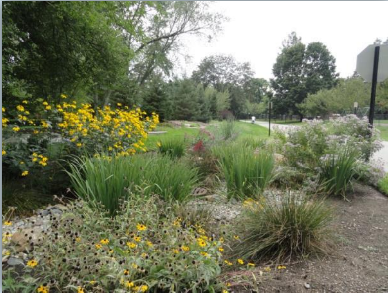
Bloomfield Hills, MI – Rain Gardens installed in 2010 to intercept storm water from road
