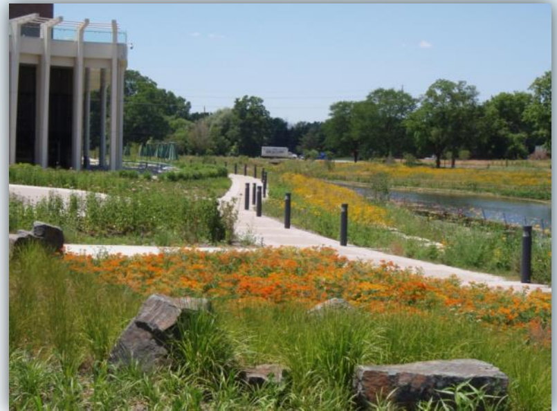
Okemos, MI – Rain Gardens and bioswales installed in 2010 to intercept storm water from parking lots and roads
