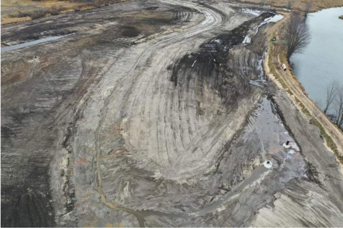
Photo 1. Sand and Gravel Bottom Post-Excavation
