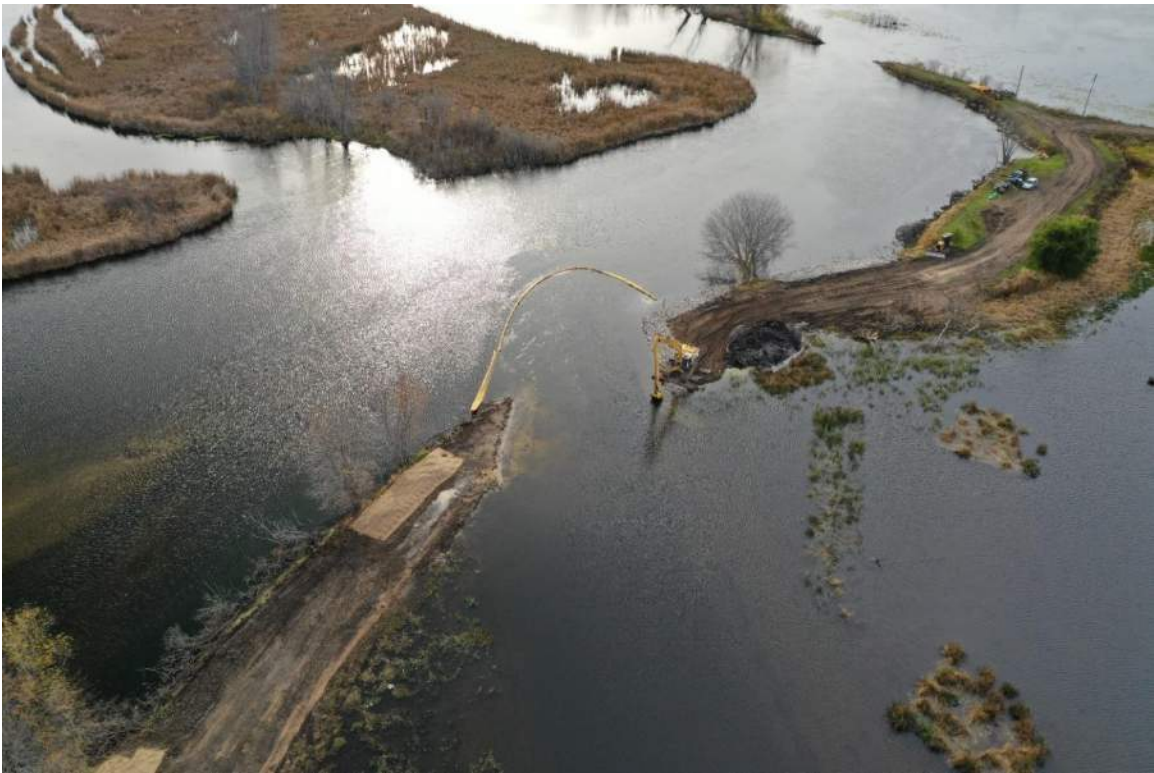
Photo 7. Berm Removal
