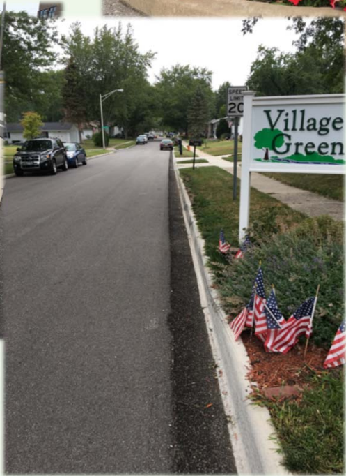
Village Green Permeable Pavement
