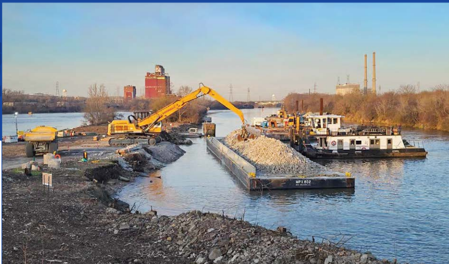
Rock excavated from the river channel for construction of the Brandon Road Interbasin Project near Joliet, Illinois, is unloaded from a barge and placed into trucks for use in another area of the project. Photo ©U.S. Army Corps of Engineers, Rock Island District.
