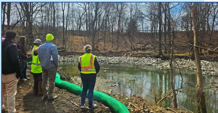
Construction work on the Jermain Park Ottawa River Restoration project in Ohio's Maumee Area of Concern (AOC), which was completed in September 2025.
