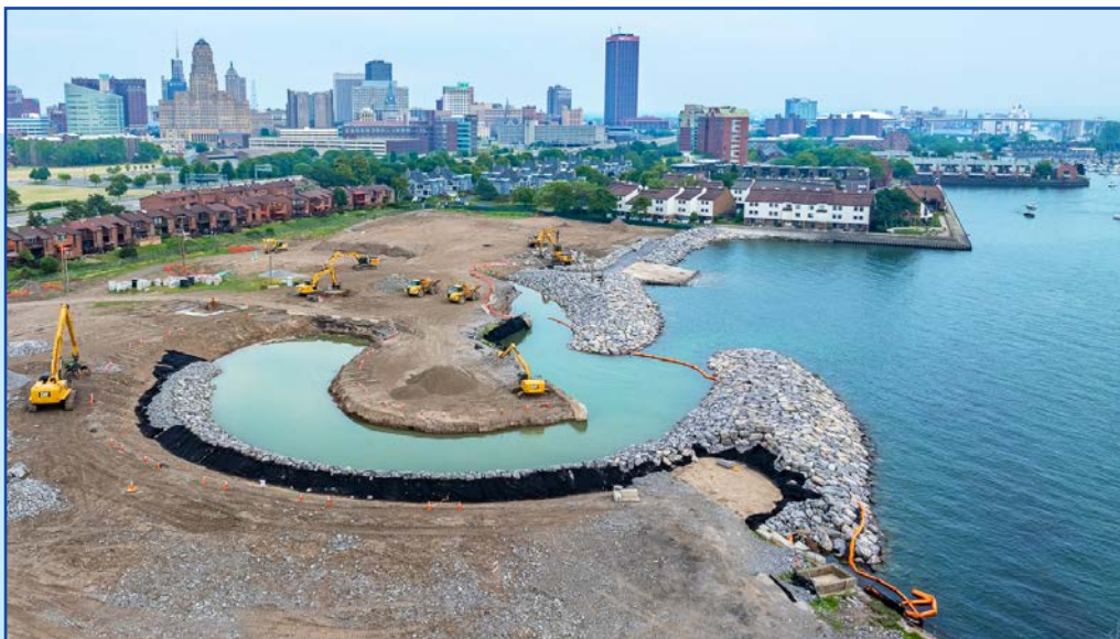
Restoration work is progressing on the transformation of Ralph Wilson Park in the Niagara River Area of Concern (AOC) in Buffalo, New York. This restoration will expand accessible recreation just steps from downtown Buffalo while supporting a more sustainable, resilient Lake Erie shoreline.
