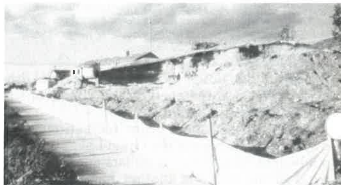
Silt fence: construction site erosion control measure. Credit: University of Wisconsin-Extension
