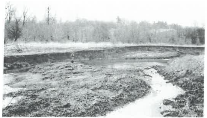
Tributary of Fox River impacted by cattle grazing and accelerated erosion. Credit: Brown County Land Conservation District (WI)
