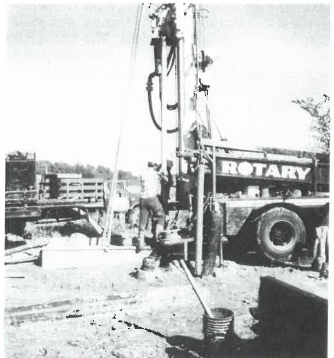
Drilling a monitor well at a landfill.
