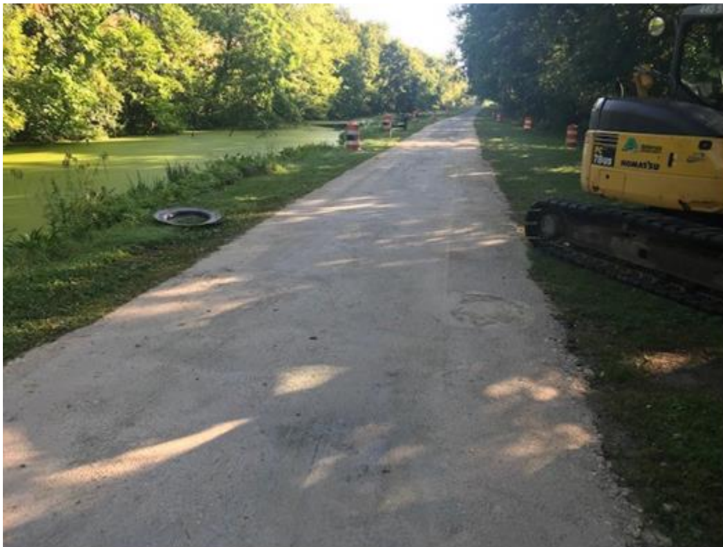
Photo 4: Minor fill and top-dressing of the towpath trail to address low spots
