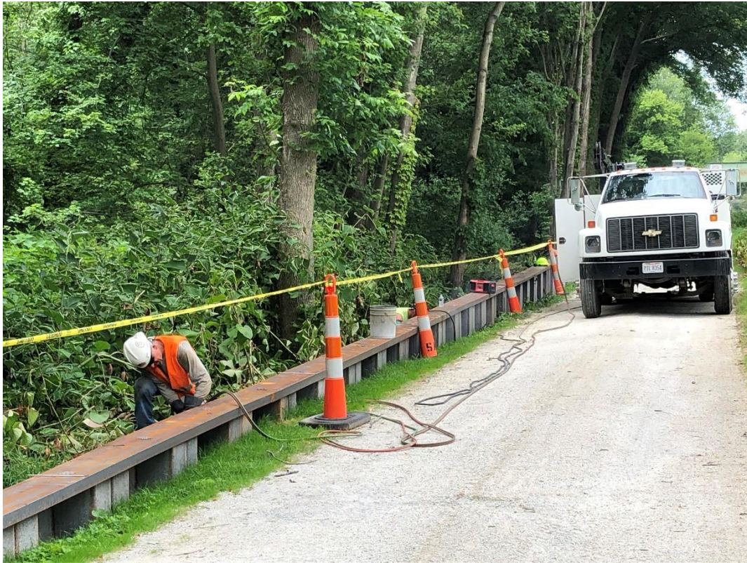
Photo 3: Steel sheet pile intended to prevent floodwater overtopping at watershed boundary
