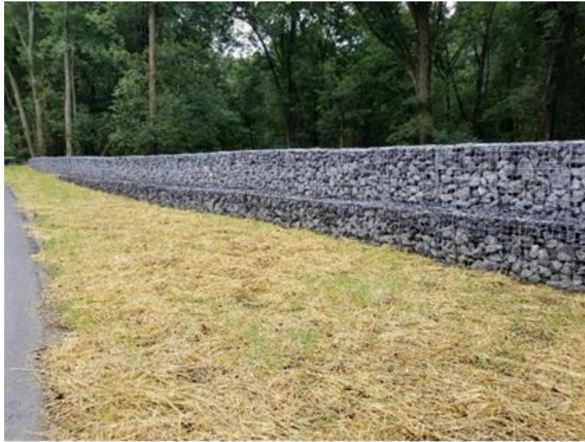
Photo 1: Gabion baskets separating floodwaters of the Great Lakes and Mississippi River Watersheds
