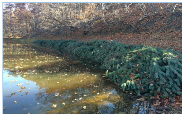
Before and after photos of one whole tree revetment installation site on the Cass River
