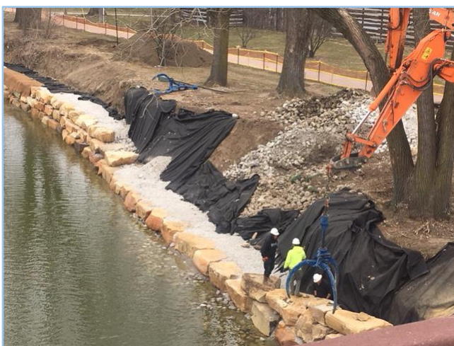
“Old Fort” bank stabilization on the St. Marys River, during construction (left) and after (right)
