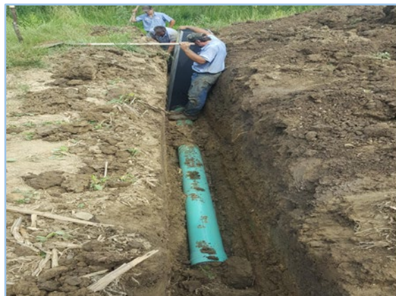
Cover crops and water control structure installation
