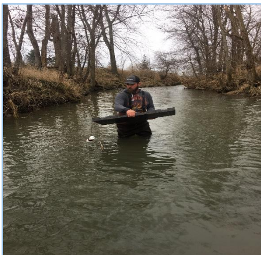
Installation of panels containing \text{PO}_4 sponge media to capture dissolved phosphorus.
