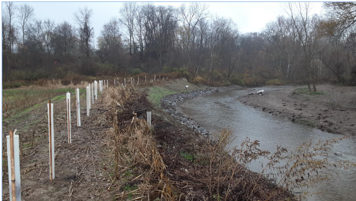
Streambank stabilization with riparian buffer plantings on Buffalo Creek in Erie County, New York.
