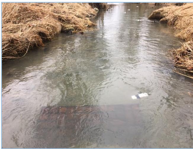
Installation of panels containing \text{PO}_4 sponge media to capture dissolved phosphorus.
