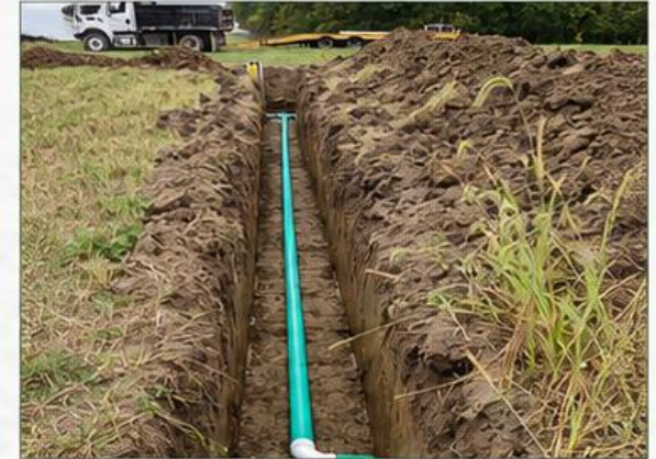
Tile drain trench
