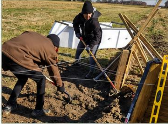
Flume installation
