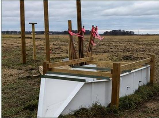
Completed surface flume
