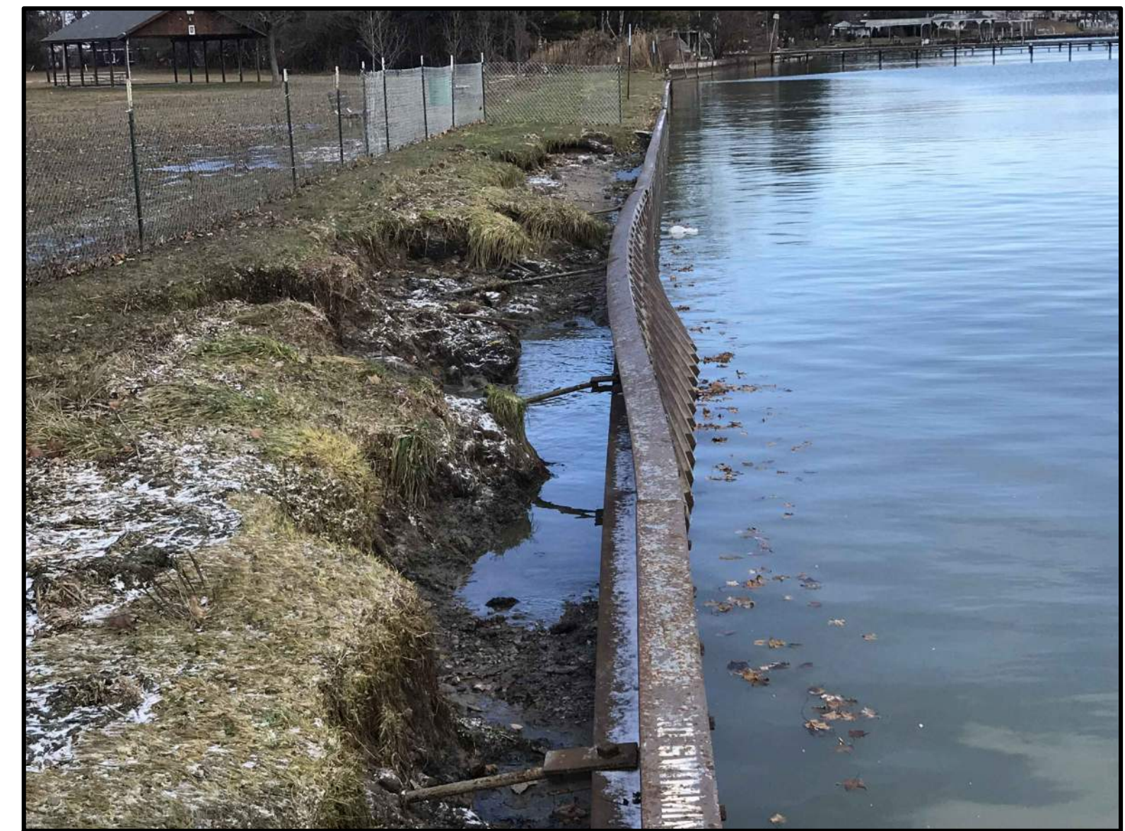
B EXISTING SEAWALL 2/12/2019
