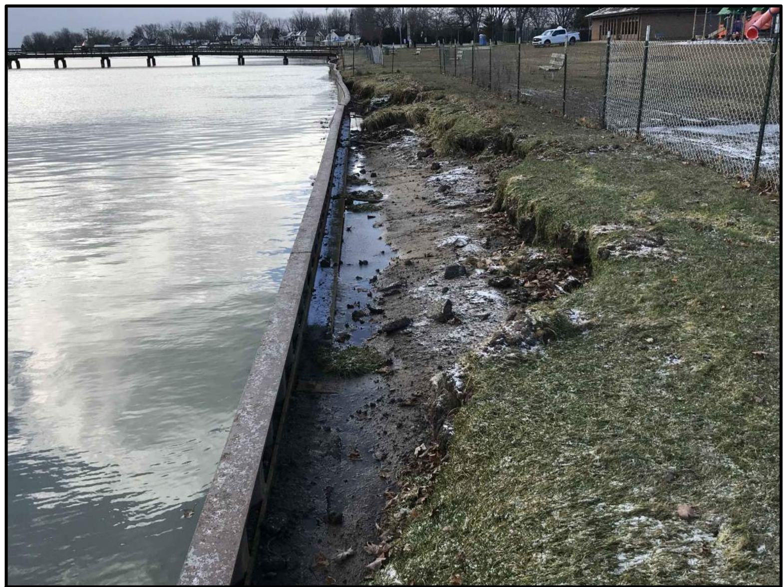
A EXISTING SEAWALL 2/12/2019
