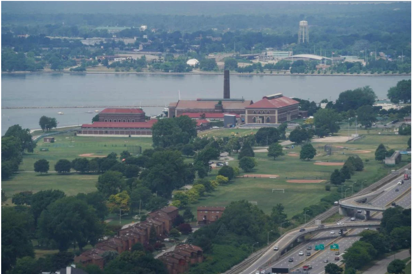
Centennial Park and the Col. Ward Pumping Station on the Niagara River in a view from Seneca One tower. Derek Gee/News file photo
