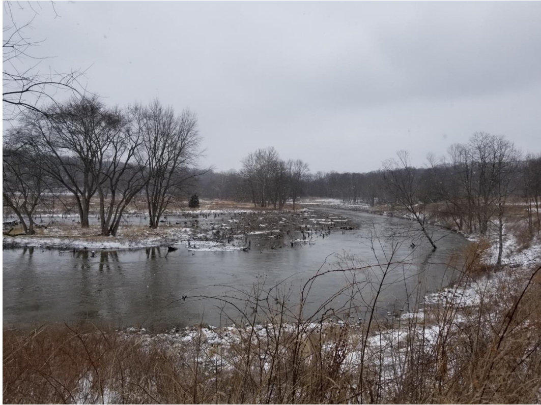
Photo 1: Flooding Event, Feb. 18 at Valley View Showing River Elevations and Debris Accumulation
