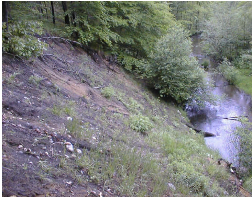
Figure 3.3.3. Area Of Significant Stream Bank Erosion Along Cedar Creek Near Sweeter Road.
