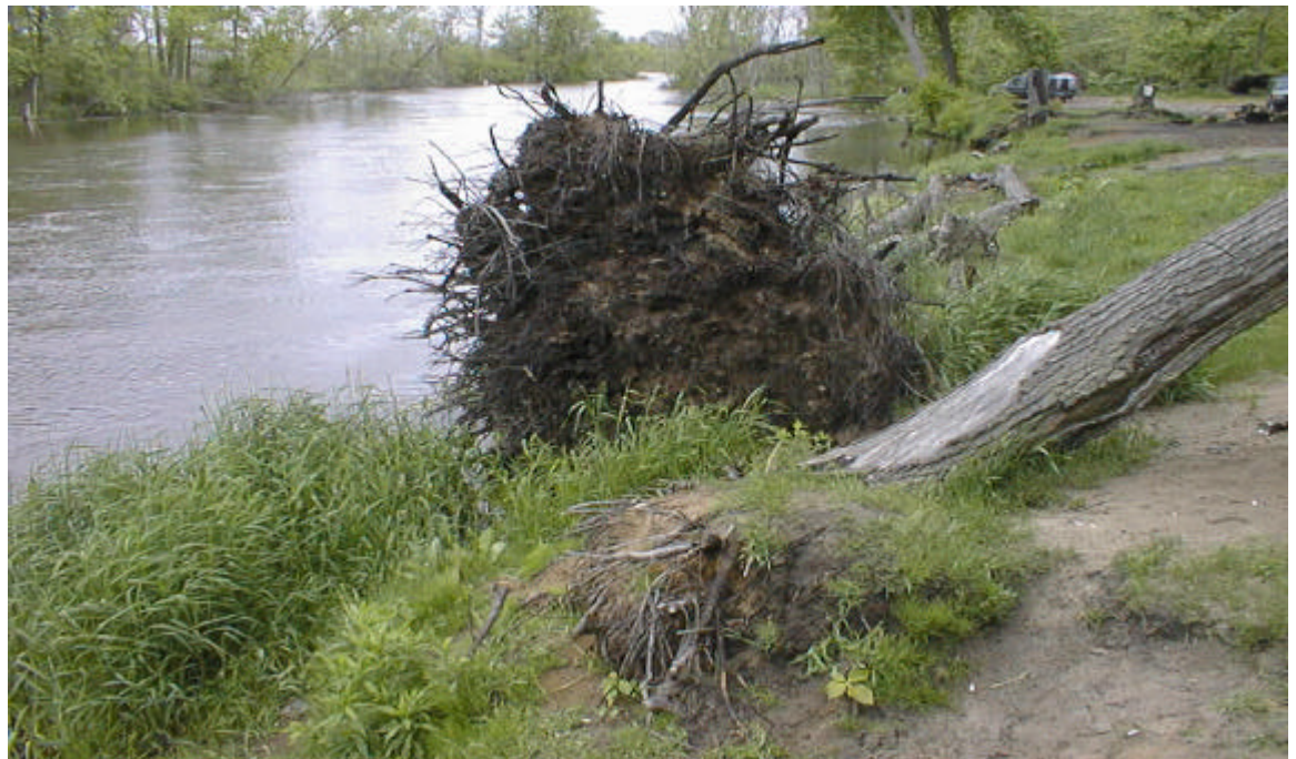
Figure C-4. Zone 2 Sheridan Road Public Access Erosional Effects
