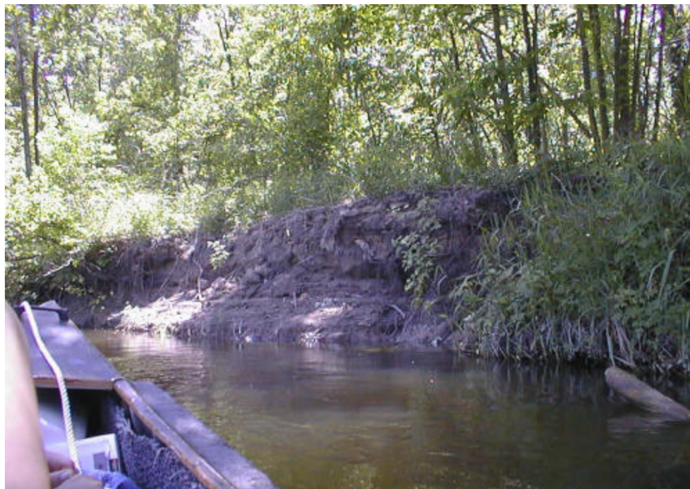
Figure 3.4.3. Typical Areas Of Erosion Within Zone 4.
