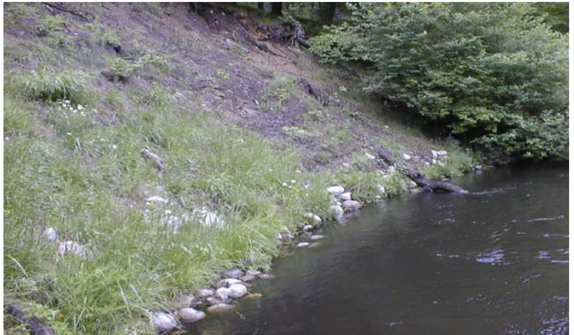
Figure C-12. Zone 3 Cedar Creek Riparian Slopes And Stabilization Projects
