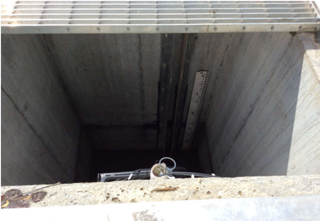
PHOTO 1: Overview of the Channel WCS on 5/27/2022.
