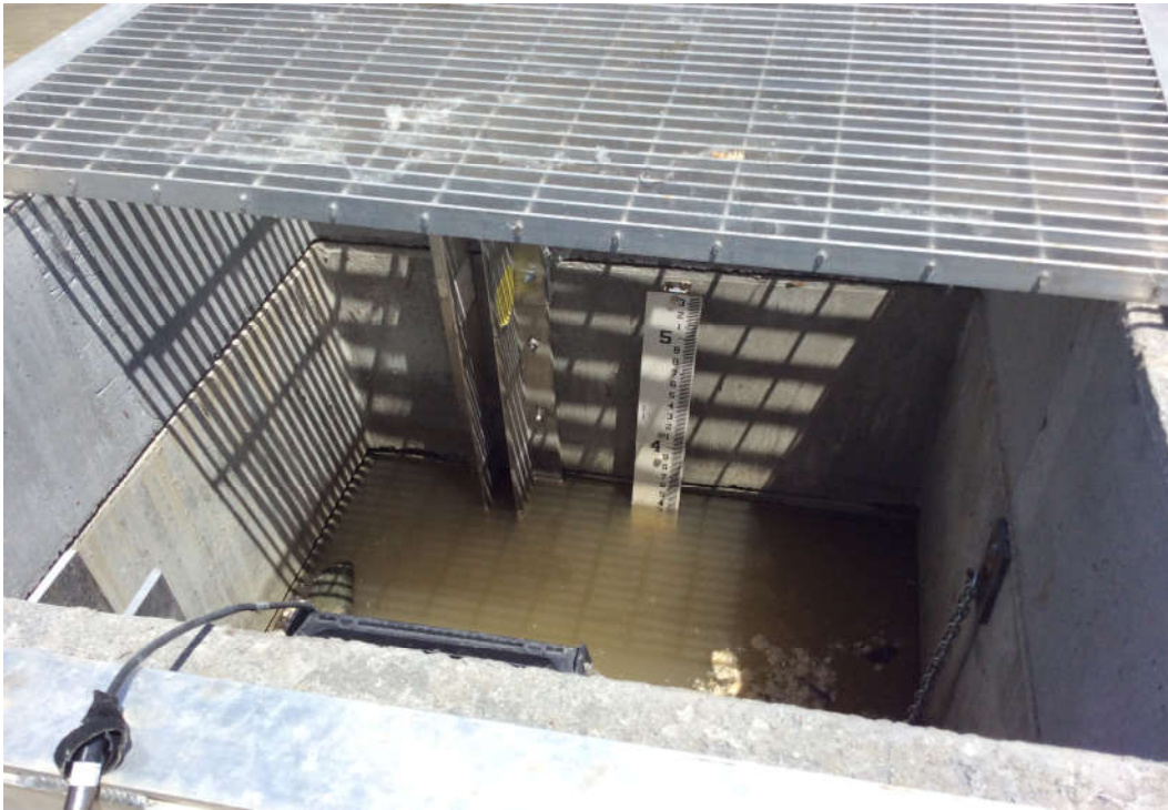
PHOTO 3: Overview of the Embayment WCS on 6/3/2022.
