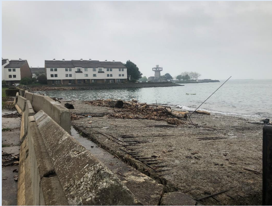
View of the hardened shoreline at the Ralph C. Wilson Jr. Centennial Park inlet area
