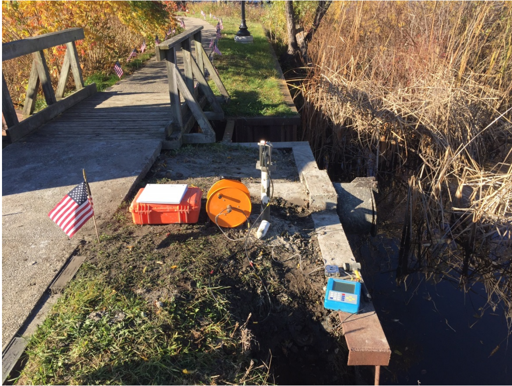
Parallel Seismic Test Setup at test location B-1
