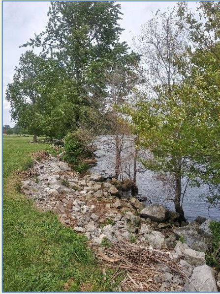
Hardened shoreline before restoration (Photo by Jill Estrada / GLC)
