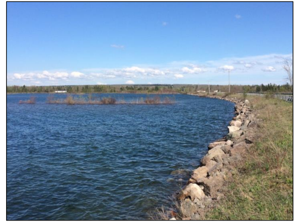
Impounded water along the Sugar Island causeway
