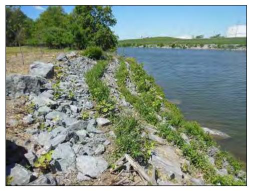
Figure 3-5. Live stakes in erosion control portion of Area 11
