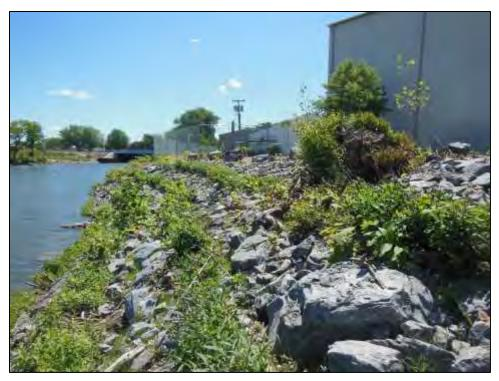
Figure 3-4. Live stakes in erosion control portion of Area 11
