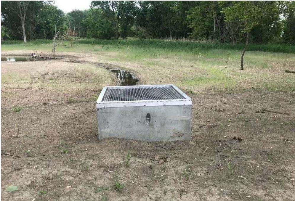
PHOTO 1: Overview of the Wetland Water Control Structure (WCS).
