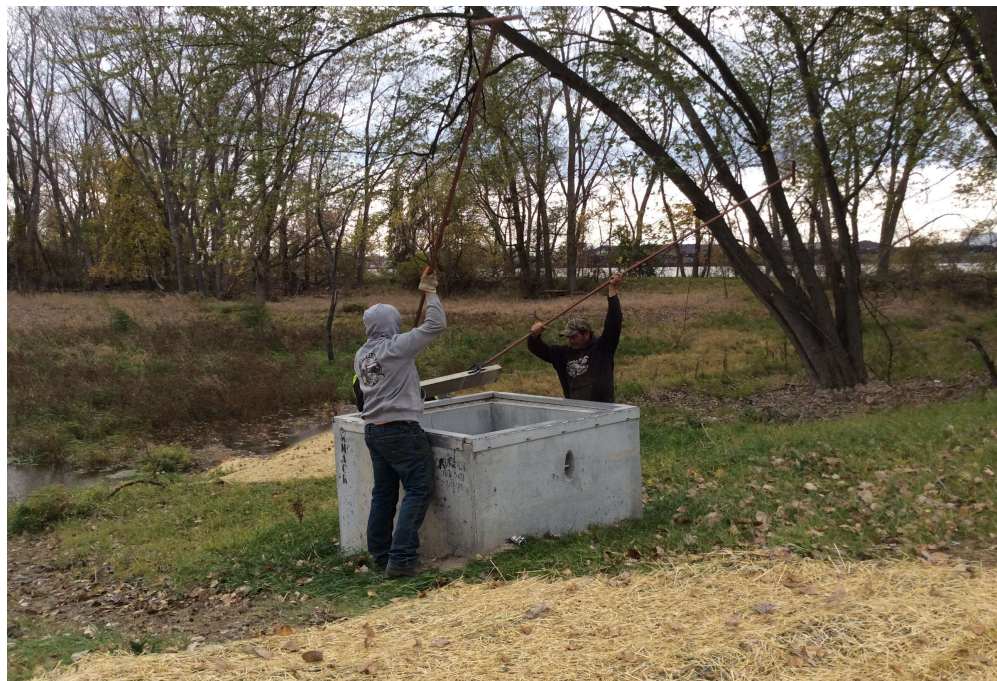
PHOTO 6: Removal of stop log from the Wetland WCS using lifting hooks.
